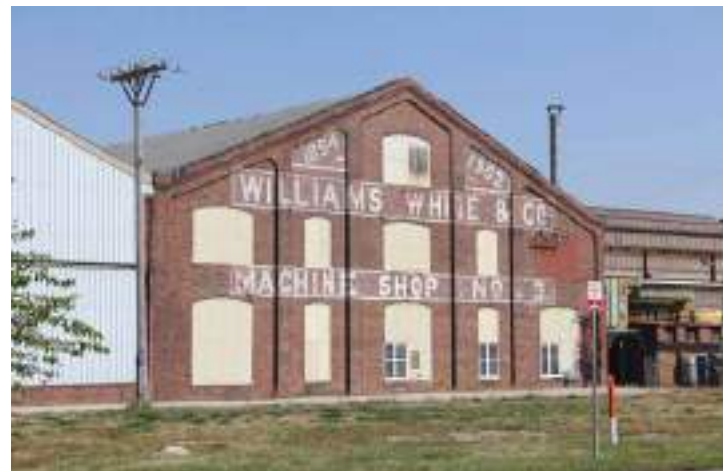
The Williams-White Company factory - viewed from Railroad Ave.
