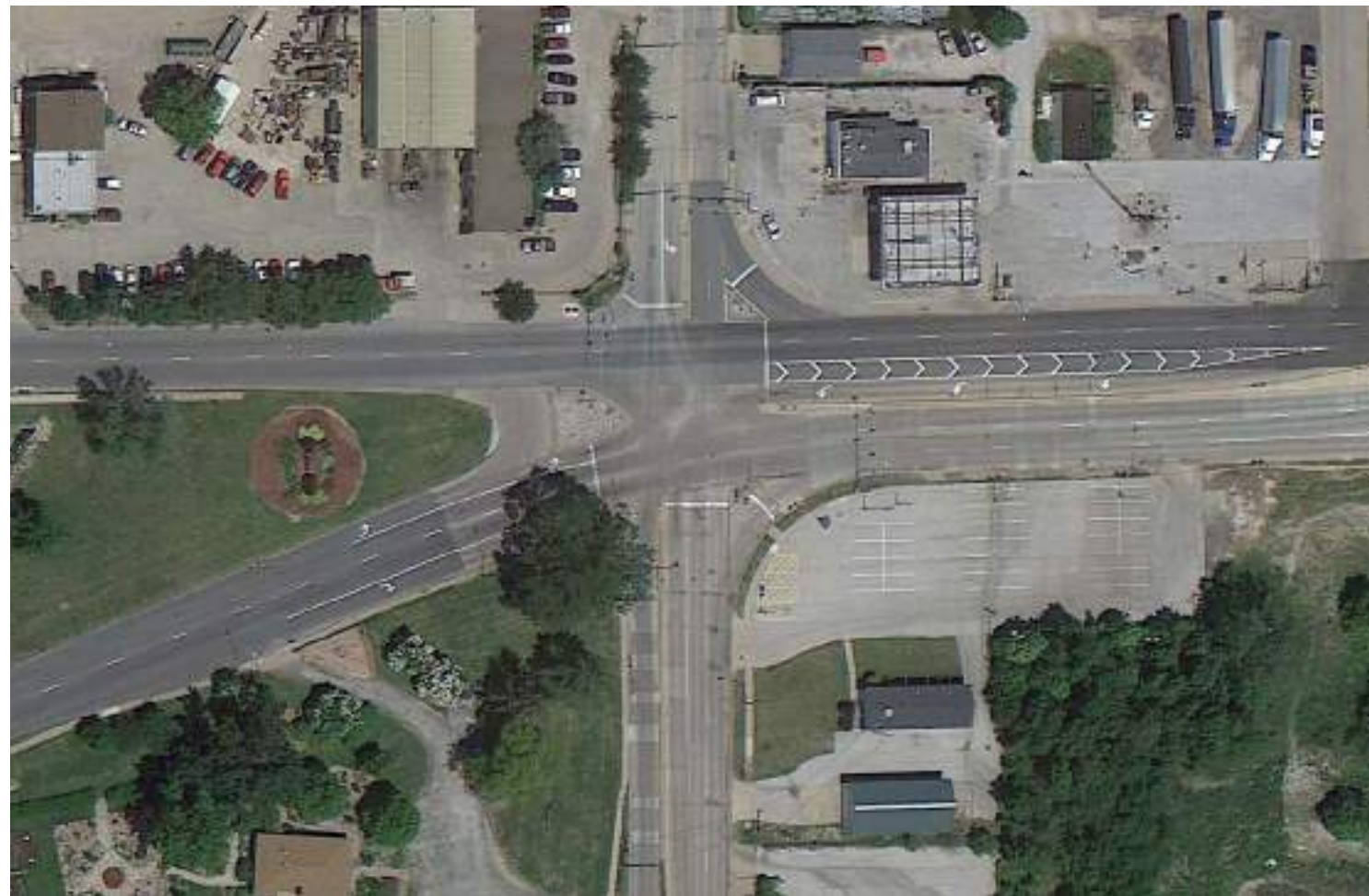
4th Avenue and 34th Street Intersection Existing Conditions
