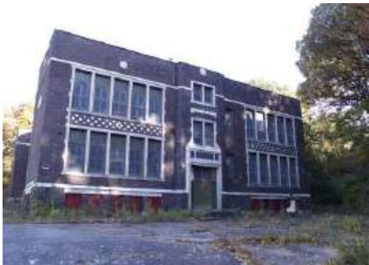
Former McKinley School at 5th Avenue and 41st Street
