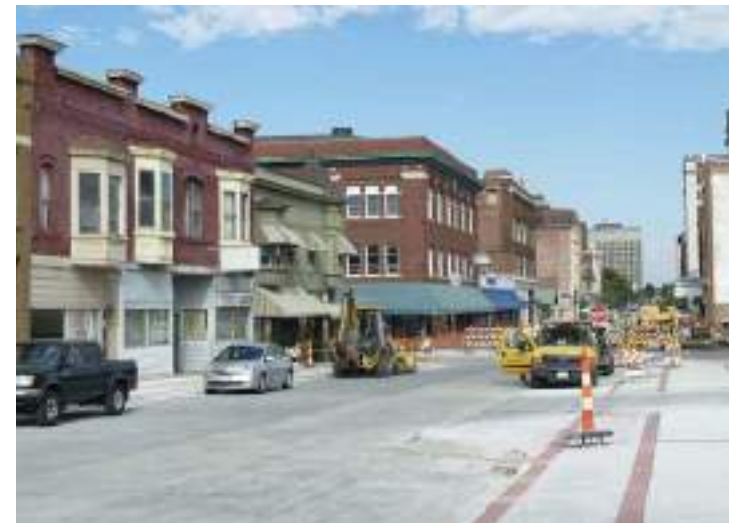
5th Avenue streetscape under construction (recently completed)
