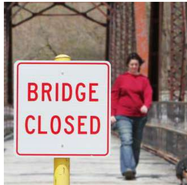
Sylvan Island Bridge is now closed to use
