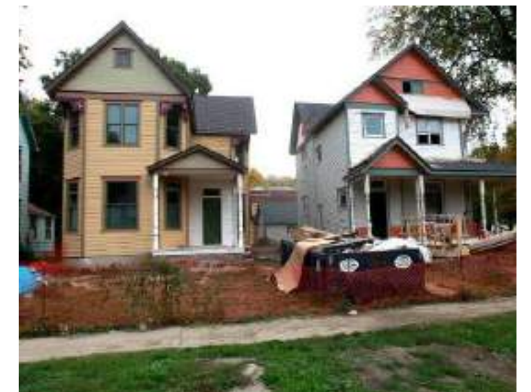
Homes under rehabilitation
