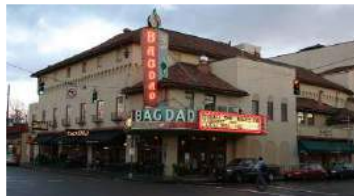
Bagdad Theatre and Pub in Portland, OR The McMenamen’s chain specializes in the adaptive reuse of historic buildings as hotels and entertainment uses.
