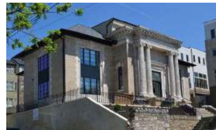
The former Carnegie Library in the Manayunk neighborhood in Philadelphia, was converted into seven apartments. Double-height front windows were divided to allow for two-story interior.
