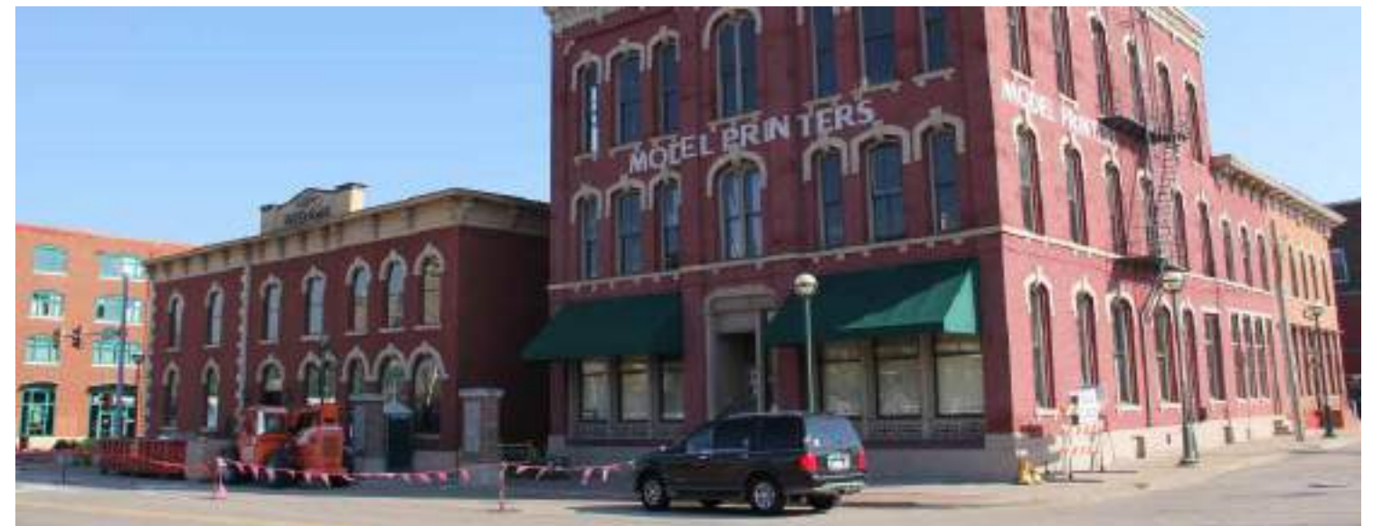
Southeast corner of River Drive at 15th Street
