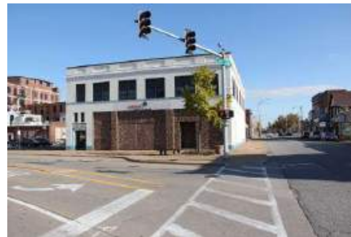
The existing building on 15th Street at 6th Avenue (see potential improvements sketch, right)
