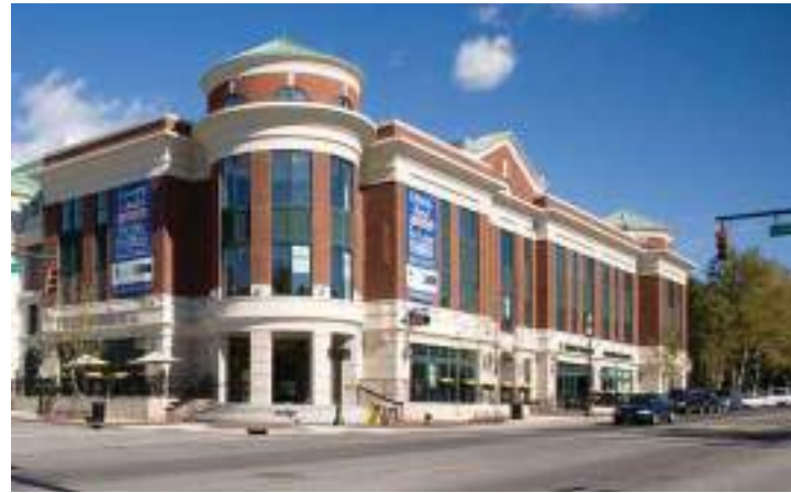
A corner entry feature provides a focal point
