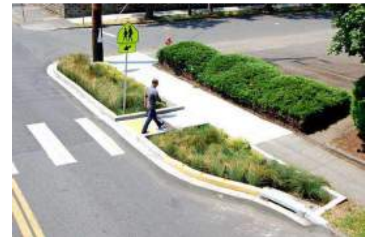
Curb extensions reduce pedestrian crossing distances
