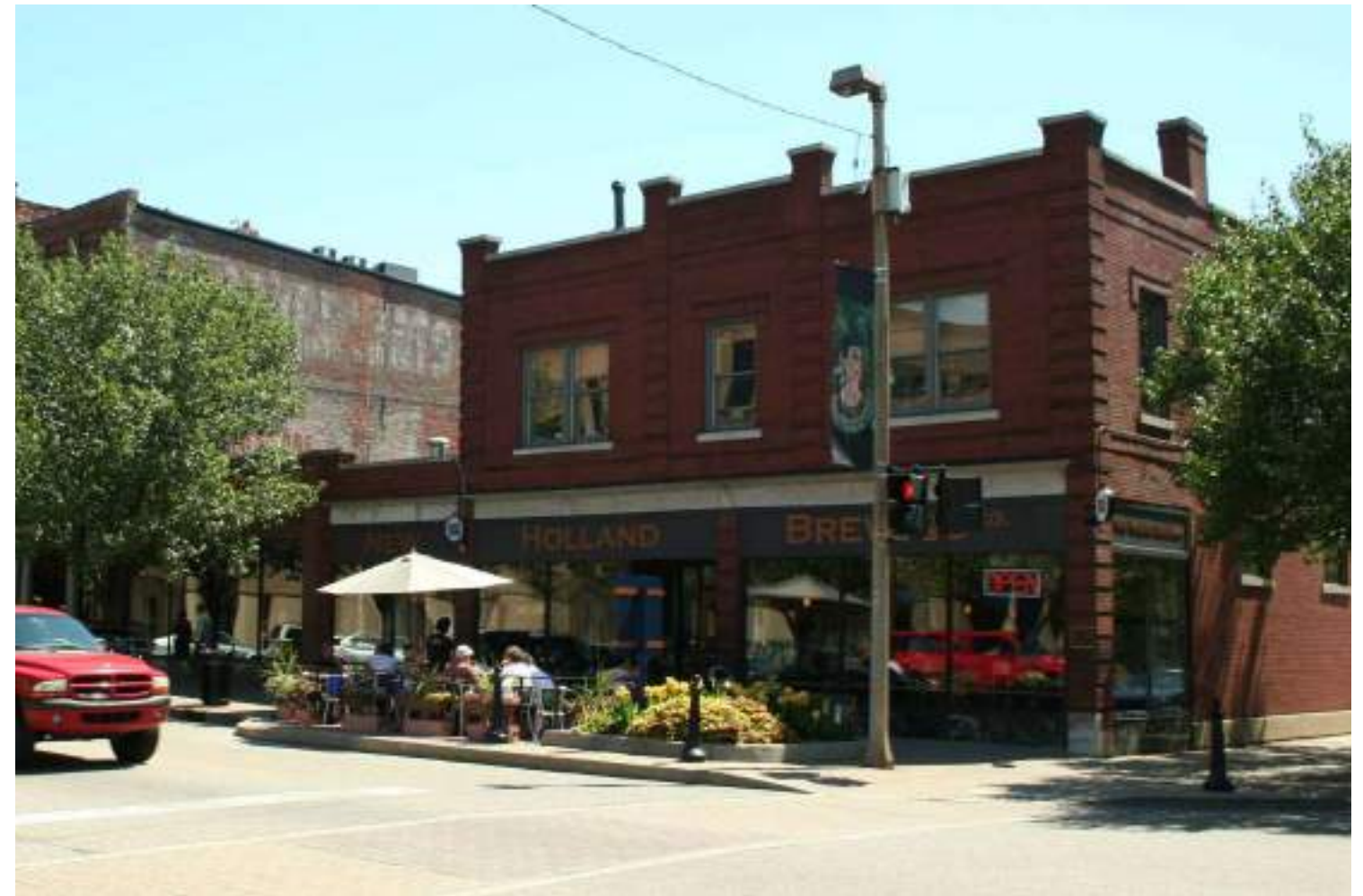
Well placed curb bump-outs can create space for outdoor dining areas and decorative landscaping.
